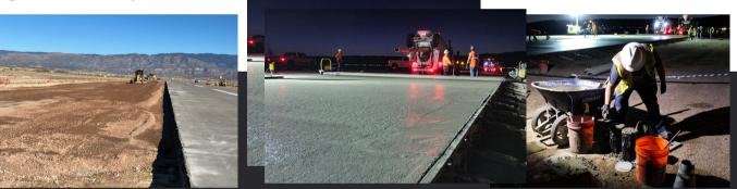
This design/build project on Holloman Air Force Base consisted of a full depth replacement of the concrete slabs in the outer two sections of the Runway 25 touchdown. We also repaired/replaced the BAK 12 arresting cable pads and foundation. All of the demolished concrete was crushed and left in the base Reuse Area. All work was completed in accordance with UFC 3-260-04, UFC 3-260-01, UFC 3-260-02, and UFC 3-353-01
